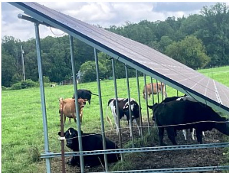
Our cows grazing under our one of our photovoltaic arrays
